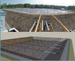
Power generation business from waste liquid from food factories (Indonesia Sumatra)
